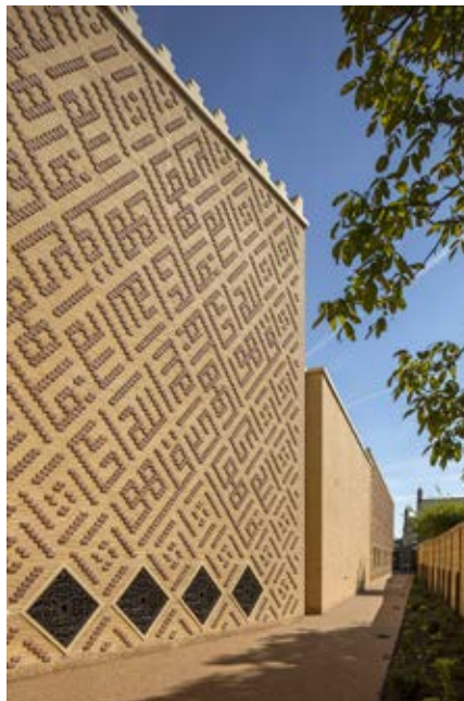
Brick tile cladding © Morley von Sternberg
