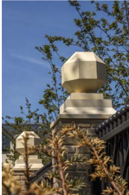
Gate post detail © Morley von Sternberg
