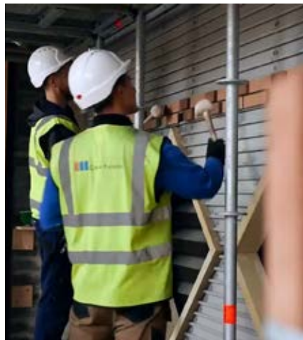
Brick tiles being clipped-in on site
