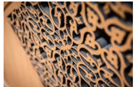
Air intake at low level with decorative fretwork © Chris Heaney
