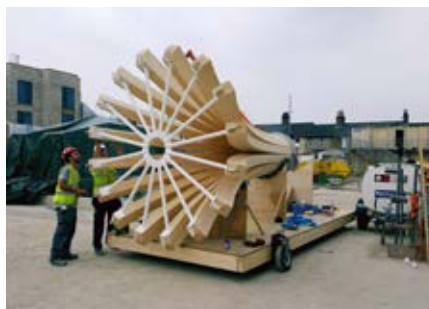
(left) September 2017 Assembly timber structure commences
